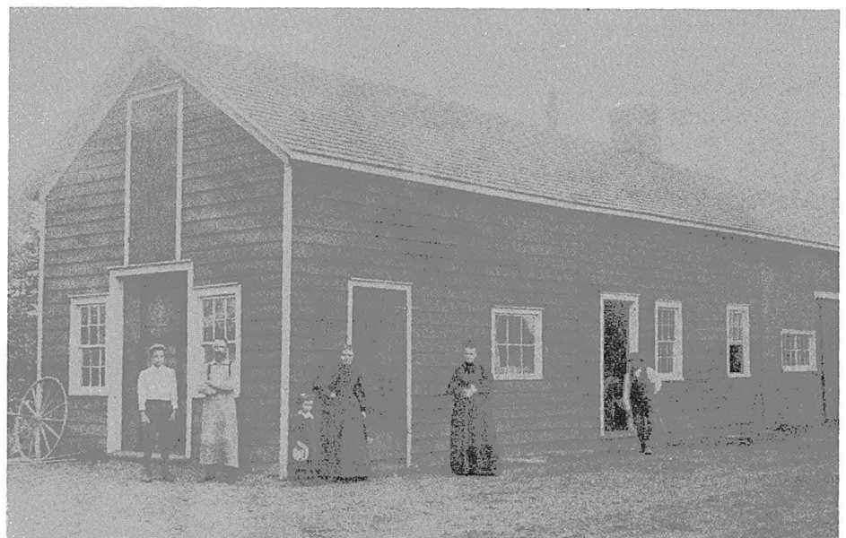
Abrams' Cooper Shop - Red Mill Road (courtesy Gerald & Annella Ingalls)
