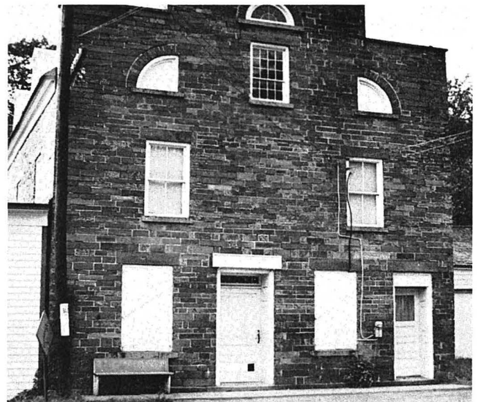
Stephens Store at Stephenville (Alcove), erected about 1808.
