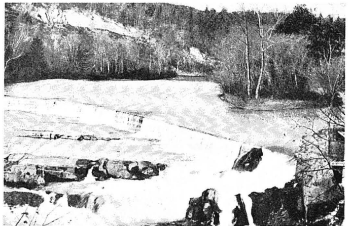
Mill Dam at Natural Dam Site, Austin's Glen
