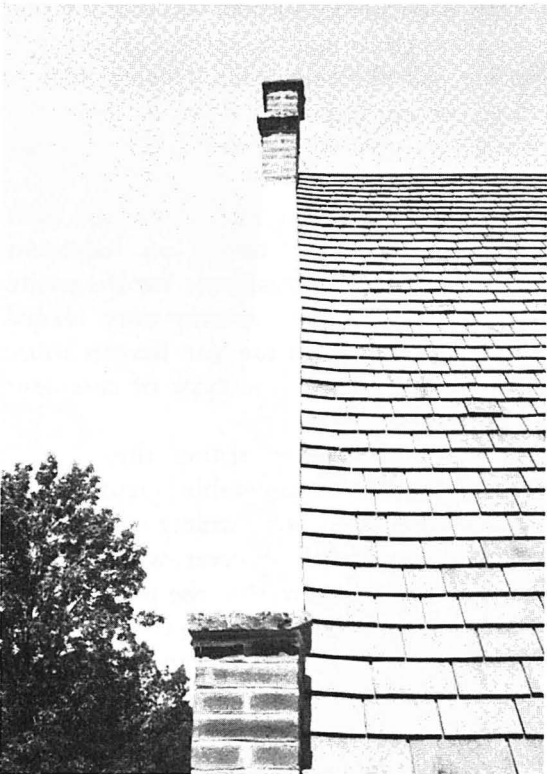
Coping on Gable parapet wall and relaid North West Side - and kneeler 1738 house.
